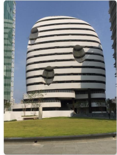
Solicitude Building (Also called Care Building)
