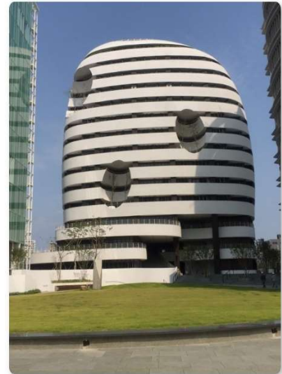
Solicitude Building (also called Care Building)
